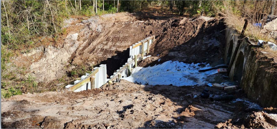
Photos at the start of the repair
