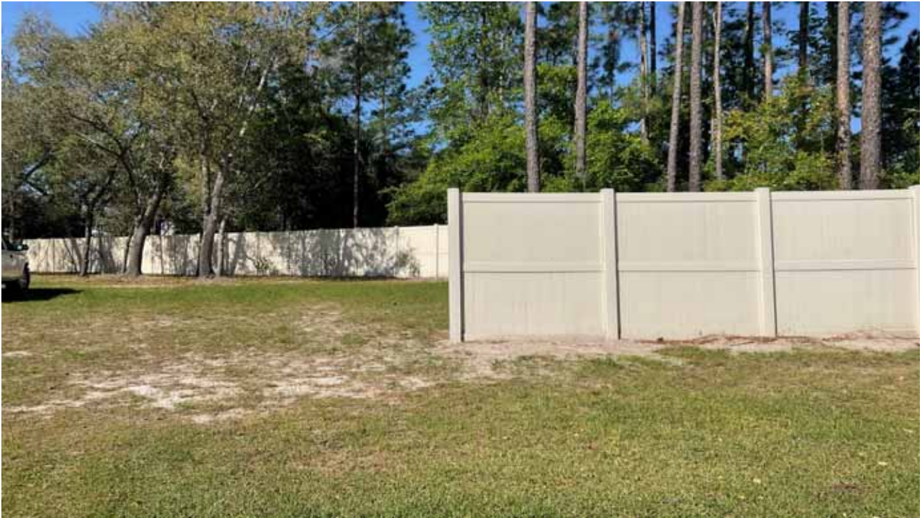
Fence - Russell Bridge Drive
