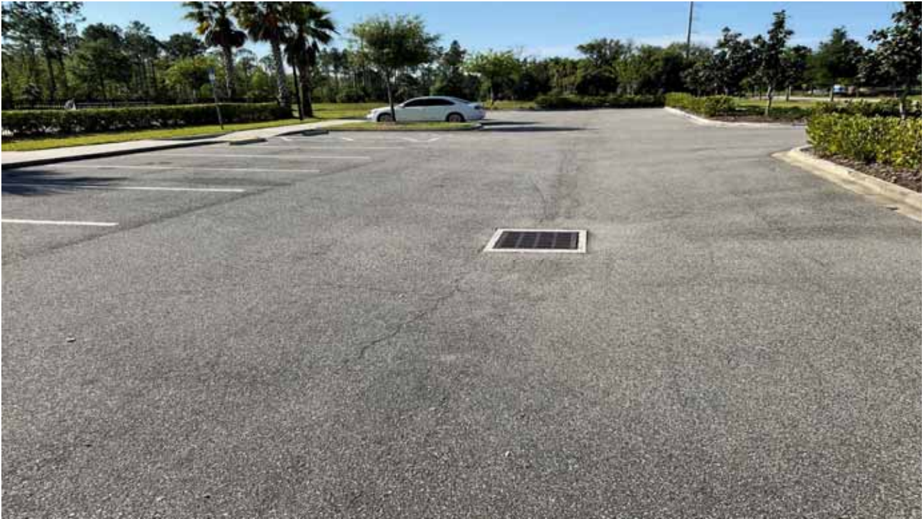
Asphalt Parking Lot
