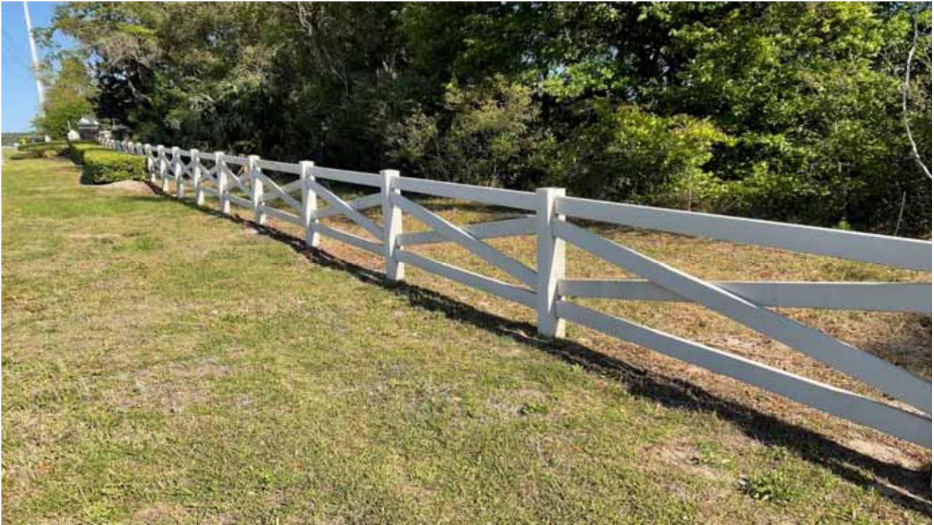
Fence - Race Track Road
