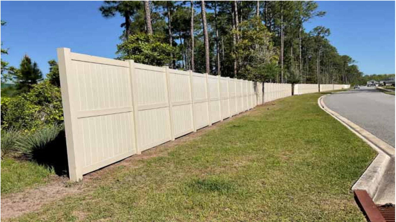
Fence - Russell Bridge Drive
