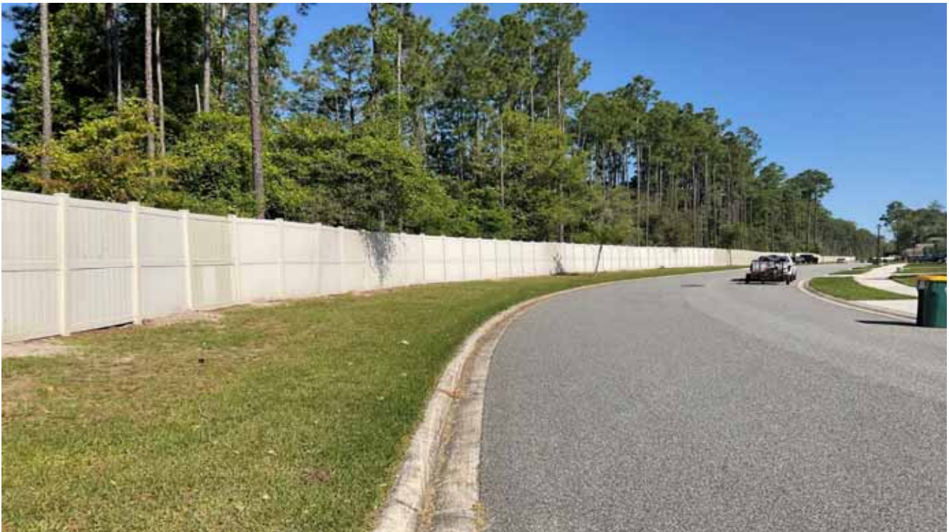
Fence - Russell Bridge Drive
