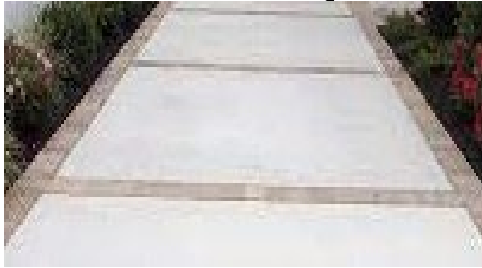
Concrete and Paver Grid
