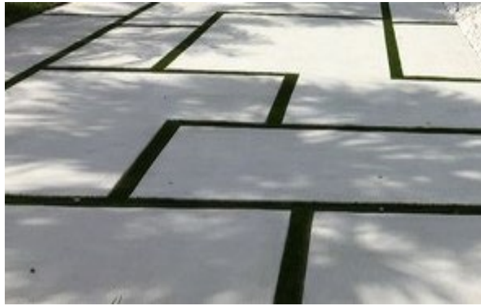
Concrete Pattern with Faux-Grass
