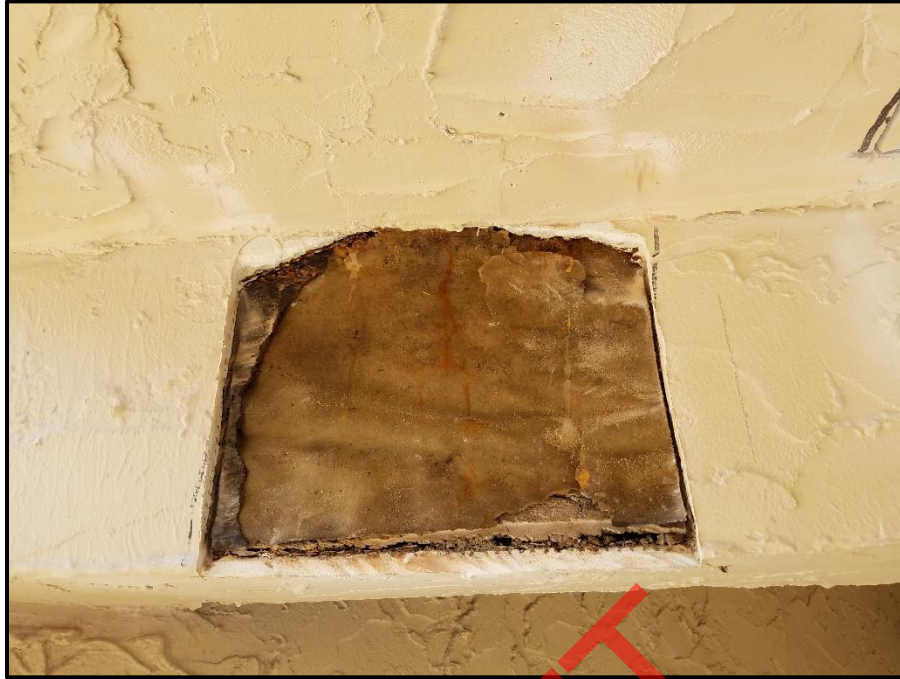
Photograph 67: Unit #301 Observation hole cut in stucco at Structural I beam.
