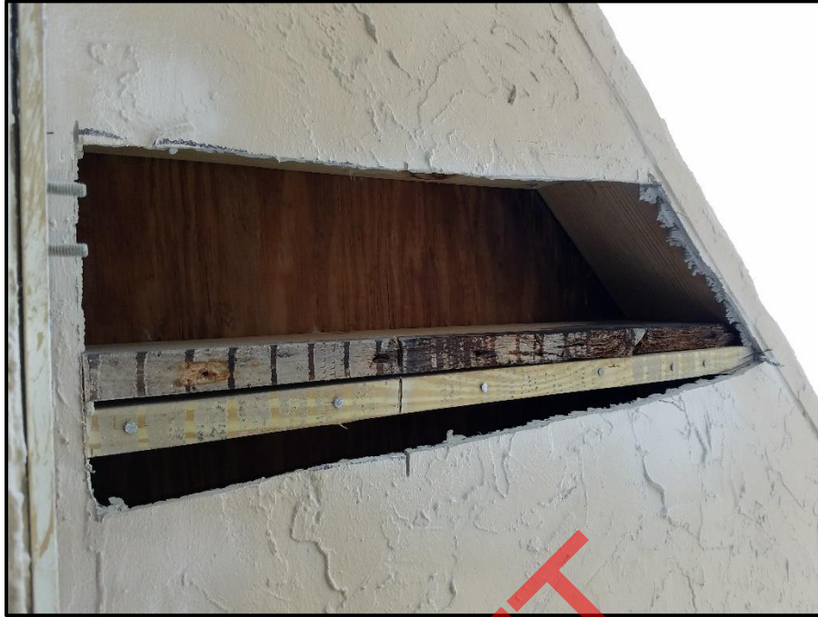
Photograph 71: Unit #303, Observation hole cut at ceiling.
