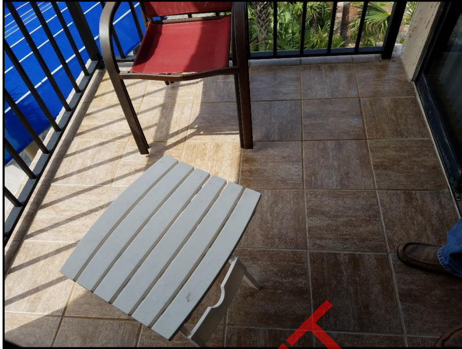
Photograph 27: Unit #402, Perspective view of balcony with tile.
