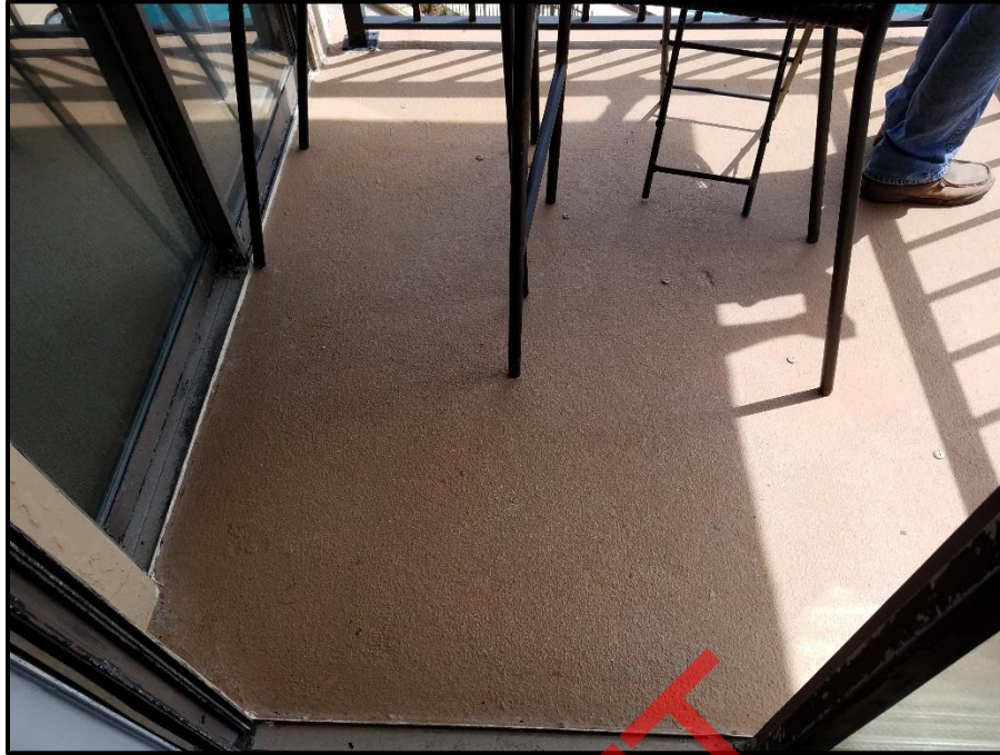
Photograph 35: Unit #403, Perspective view of balcony.
