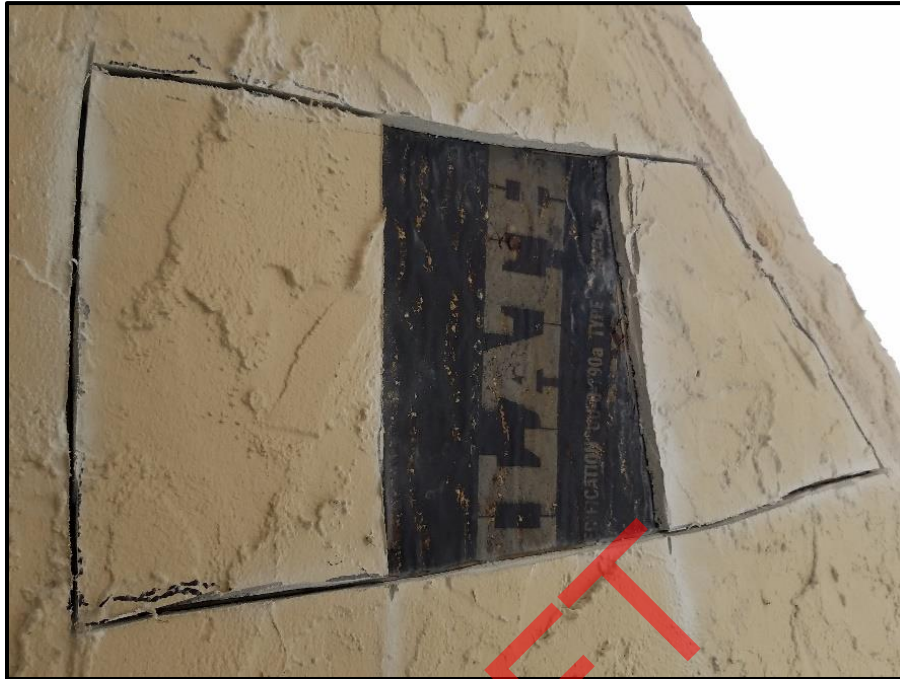
Photograph 15: Unit #204, Observation hole cut in stucco ceiling.
