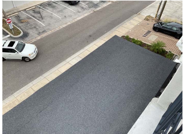
Modified bitumen roof at front elevation balconies
