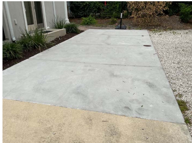
Recently replaced section
