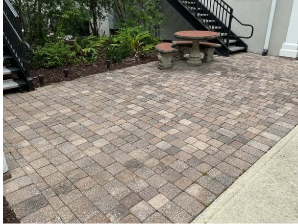
Pavers at staircase landing
