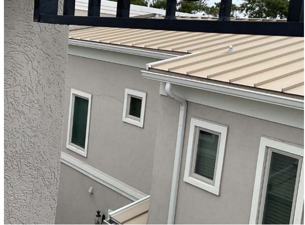
Stucco cracks
