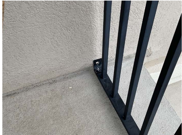
Mechanically attached railing
