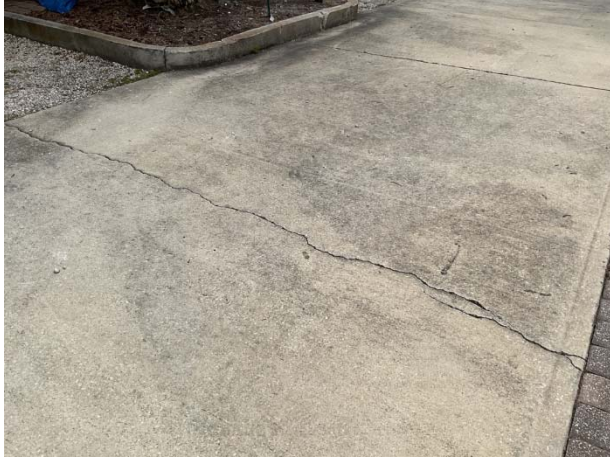
Driveway cracks
