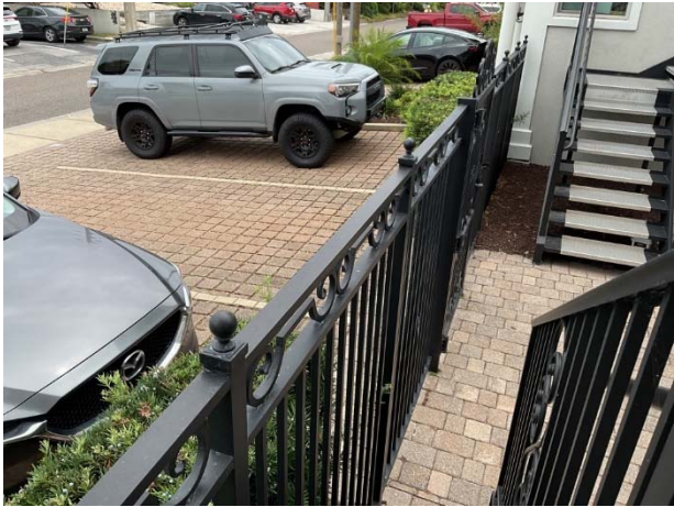
Aluminum fence at courtyard
