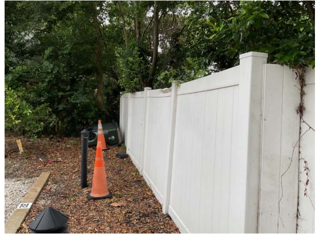
Fence panel damage
