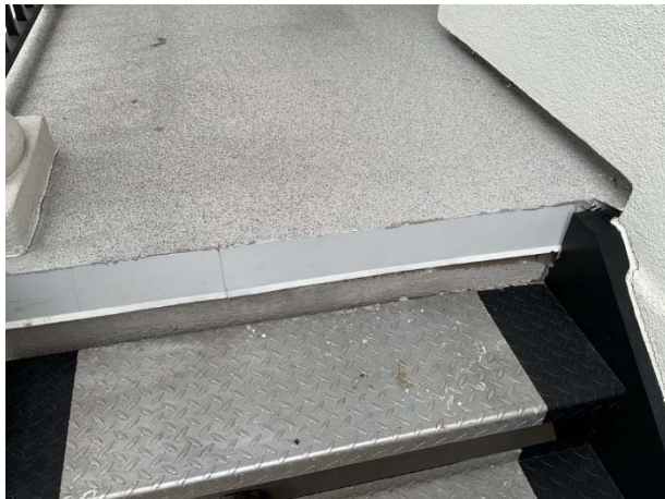
Flashing at breezeway perimeter
