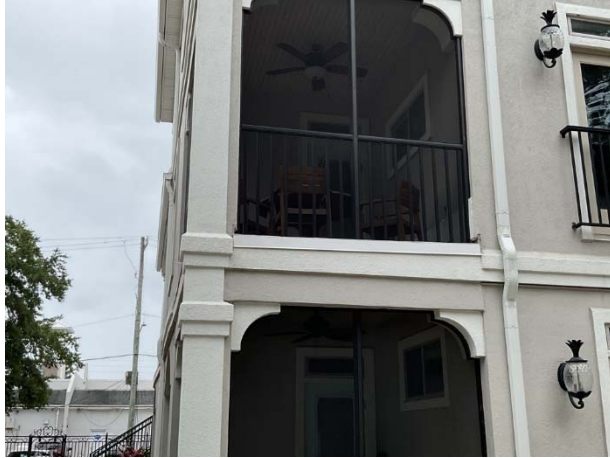
Balcony surfaces sloped away from structure
