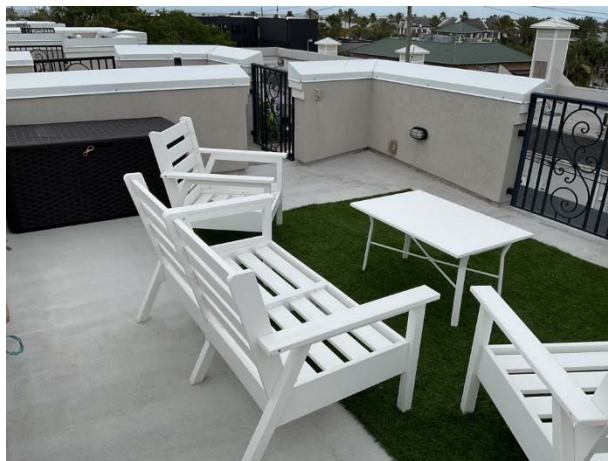
Rooftop terrace overview
