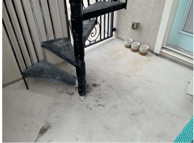
Wood frame balcony with concrete surface
