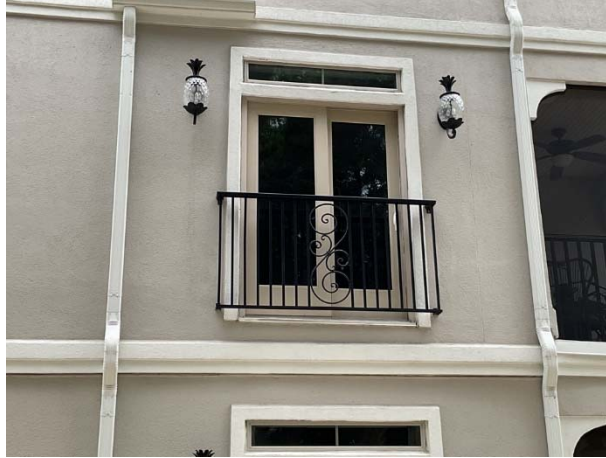
Decorative railings at Juliet balconies
