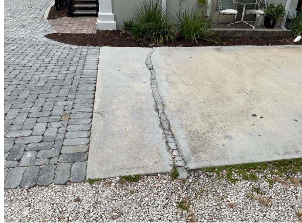
Spalled concrete
