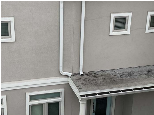
Downspouts discharging onto lower roof section
