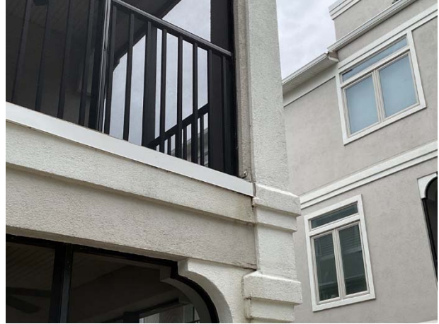
Flashing and diverter at balcony
