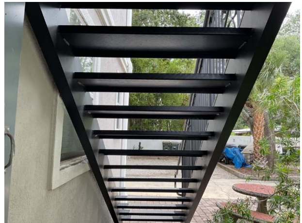
Metal staircase structure
