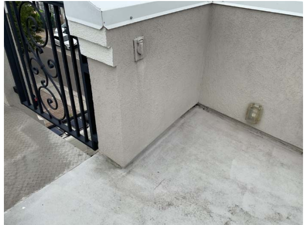
Stucco terminates above terraces
