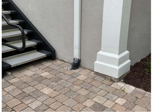
Downspout directed into drain
