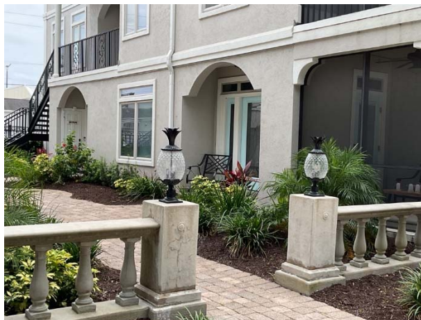
Light fixtures at courtyards
