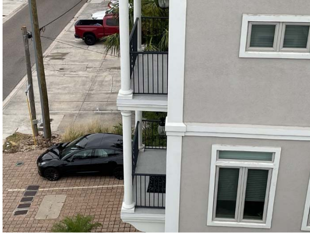
Wood frame balconies with concrete surfaces overview
