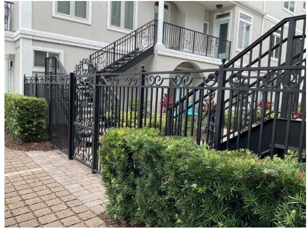
Aluminum fence at courtyard
